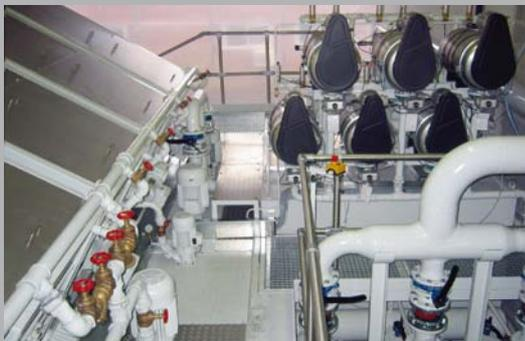
Disc-O-Filter © for fine filtration in a combined system
